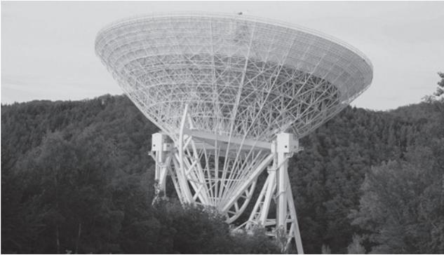
Scientists explore deep space by using large antennas to listen for distant radio waves. Parabolic antennas amplify faint signals by using the properties of parabolas to focus them onto a receiver. The worldwide Deep Space Network also helps to keep track of exploratory spacecraft like the two Voyager spacecrafts, which have left our Solar System!
