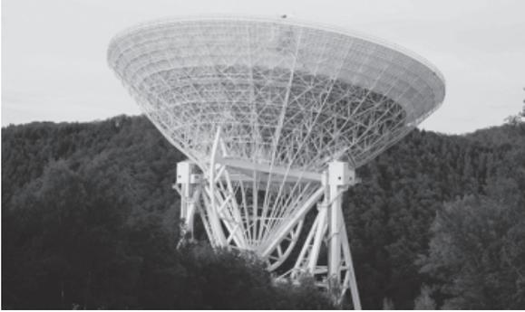
Scientists explore deep space by using large antennas to listen for distant radio waves. Parabolic antennas amplify faint signals by using the properties of parabolas to focus them onto a receiver.
